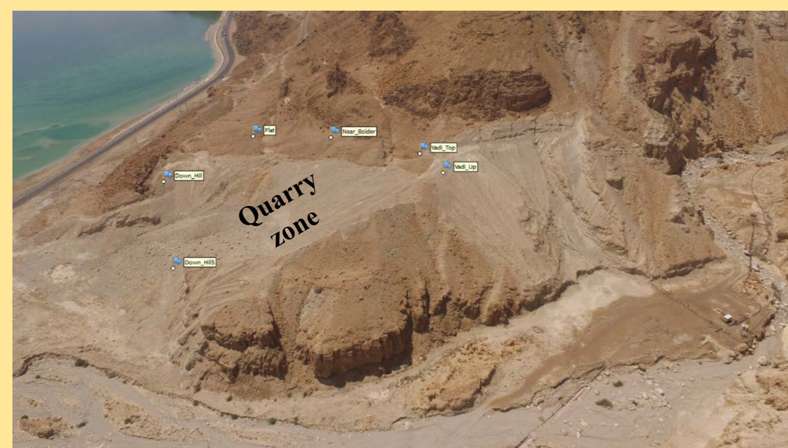
Final landmarks used to build the model
